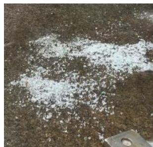
Piles of salt, shown in the photo above, are an example of a wasteful practice
