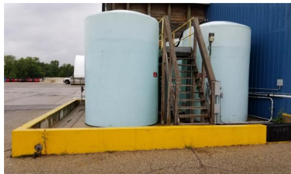
The short, concrete, wall is an example of secondary containment.
