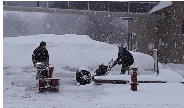
An example of a two-pass strategy: operators first use a snow blower followed by a broom.
