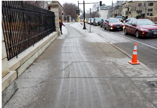
In this photo, notice the lines showing effective anti-icing application on the sidewalk.
